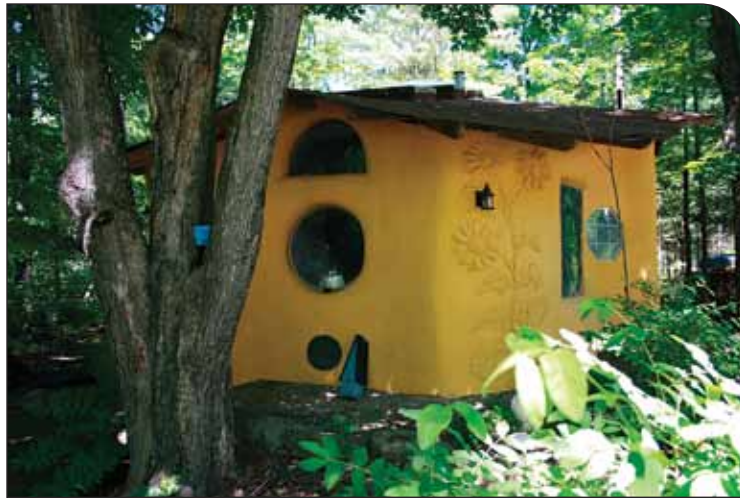
Ross and Kathryn Elliott's LEED Gold Standard home and straw bale studio in McDonalds Corners are on the Oct. 6 tour
